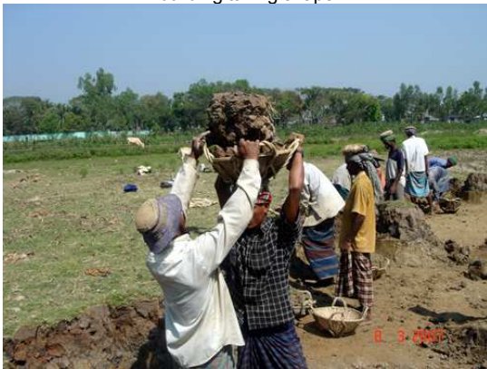
earth digging - manually
