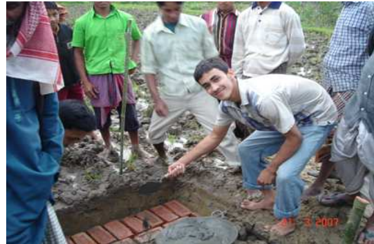
foundation laying by a volunteer
